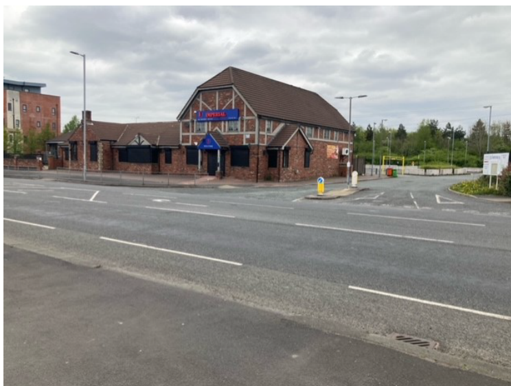
View of the existing building from Victoria Avenue East
